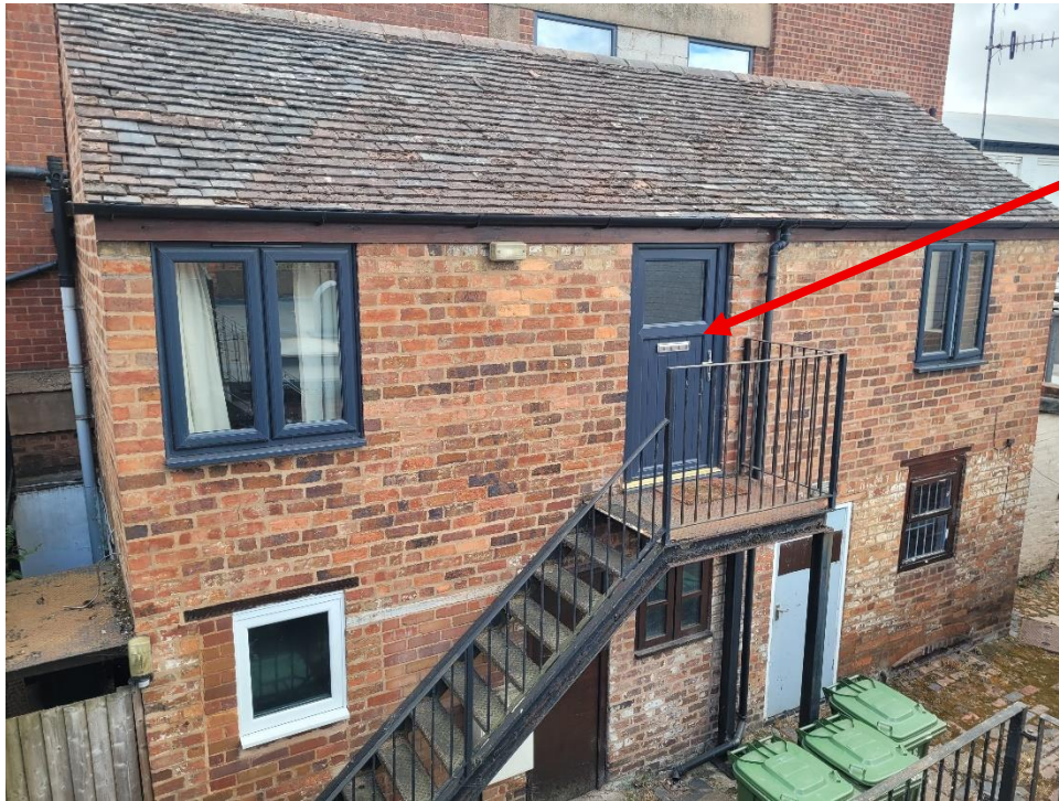
Entrance to Flat 5b – currently vacant
